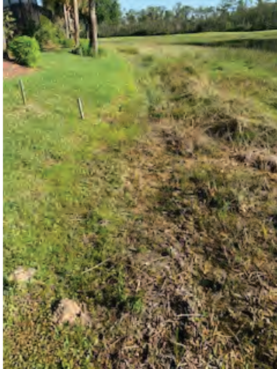
Photo 11 Minor erosion on the lake slope
