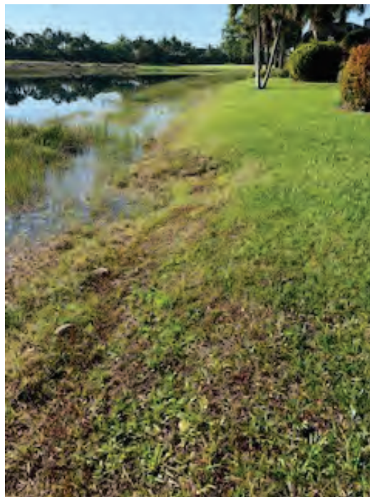
Photo 10 Minor erosion on the lake slope
