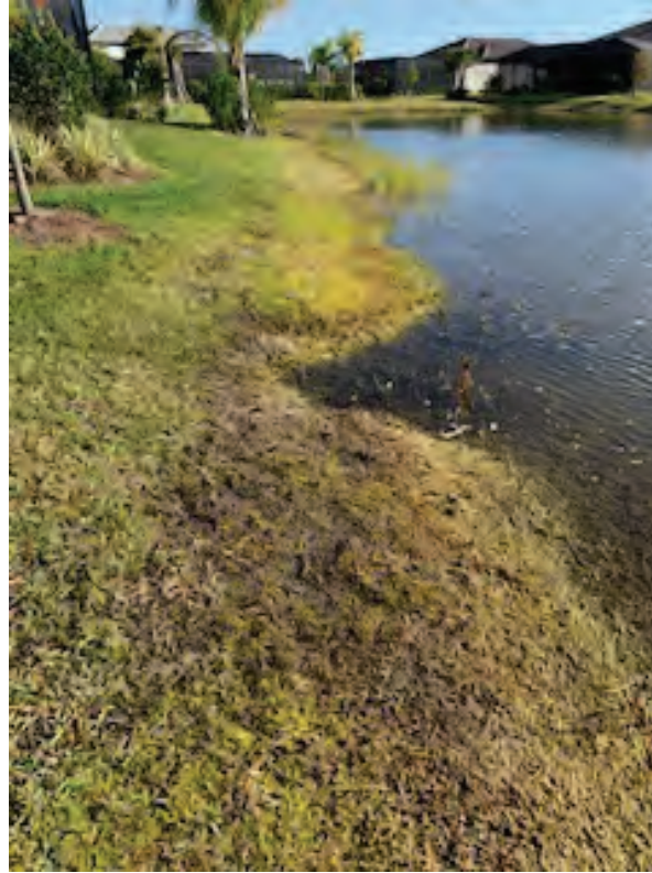
Photo 33 Minor erosion on the lake slope
