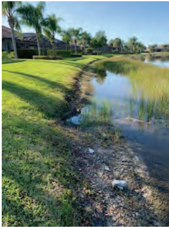
Photo 9 Minor erosion on the lake slope
