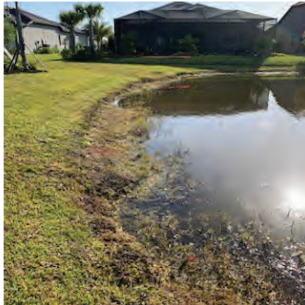
Photo 32 Minor erosion on the lake slope
