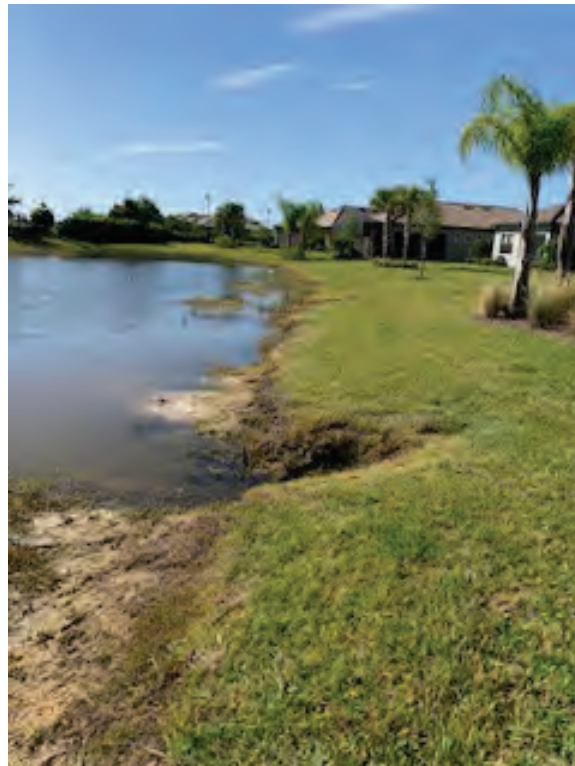
Photo 30 Extensive erosion on the lake slope
