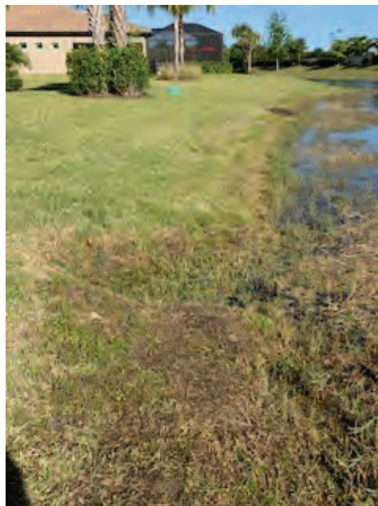
Photo 54 Extensive erosion on the lake slope
