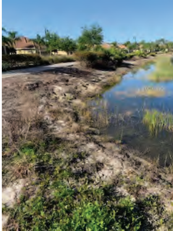
Photo 21 Minor erosion on the lake slope
