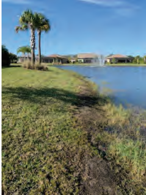
Photo 53 Minor erosion on the lake slope
