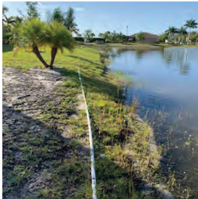
Photo 34 Minor erosion on the lake slope
