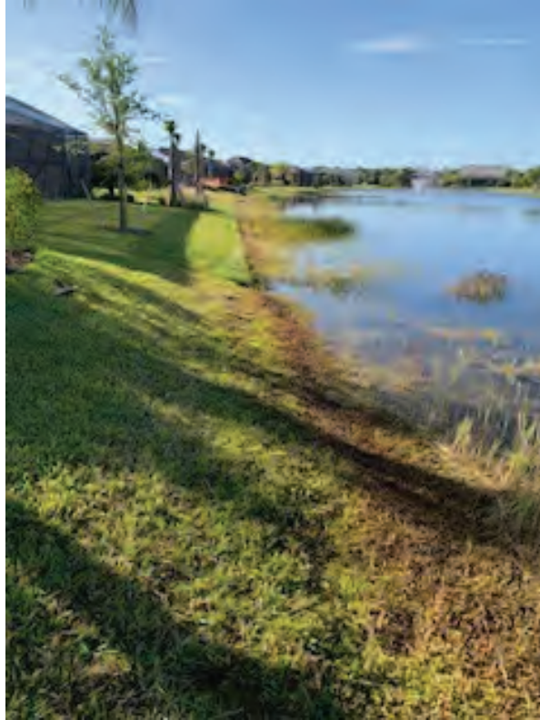
Photo 47 Minor erosion on the lake slope
