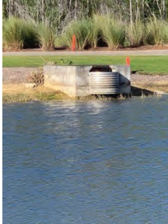
Photo 19 Minor erosion on the lake slope
