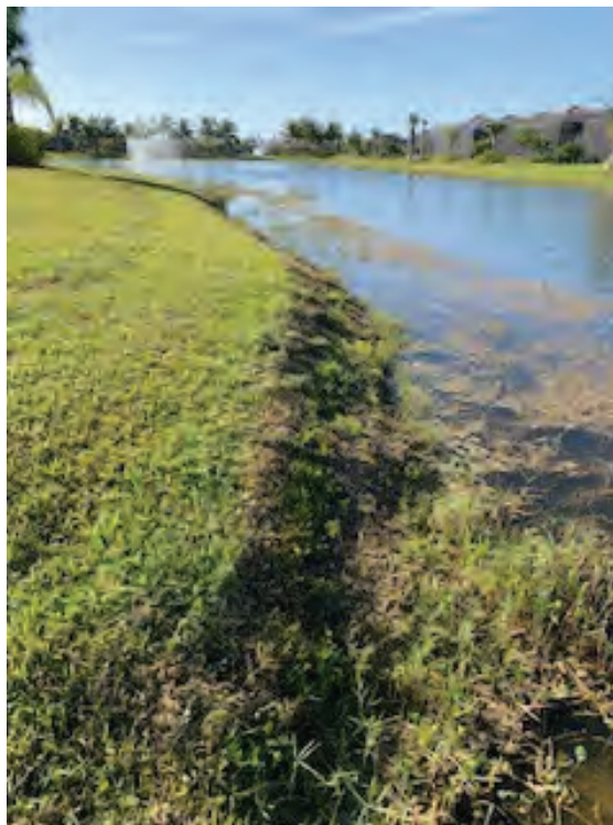
Photo 52 Minor erosion on the lake slope
