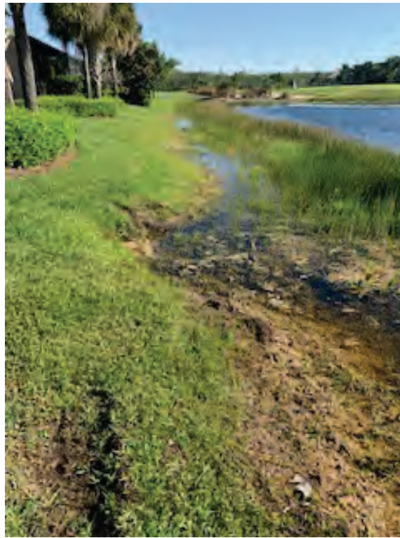
Photo 35 Minor erosion on the lake slope
