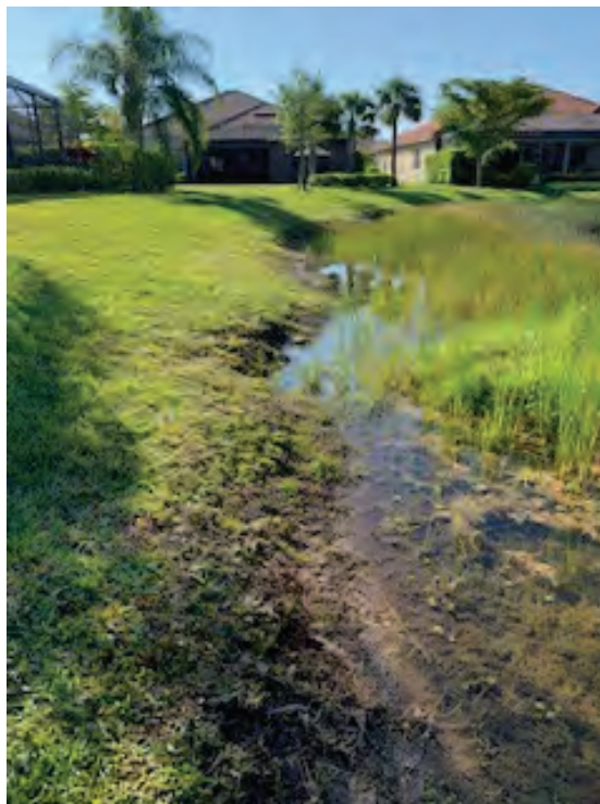
Photo 4 Minor erosion on the lake slope
