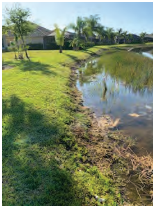
Photo 8 Minor erosion on the lake slope
