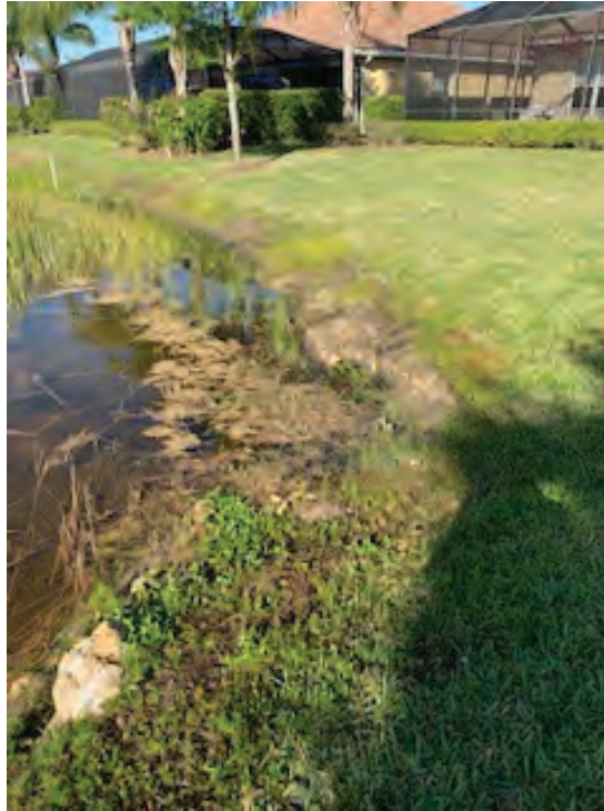
Photo 7 Minor erosion on the lake slope
