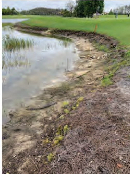
Photo 59 Extensive erosion on the lake slope
